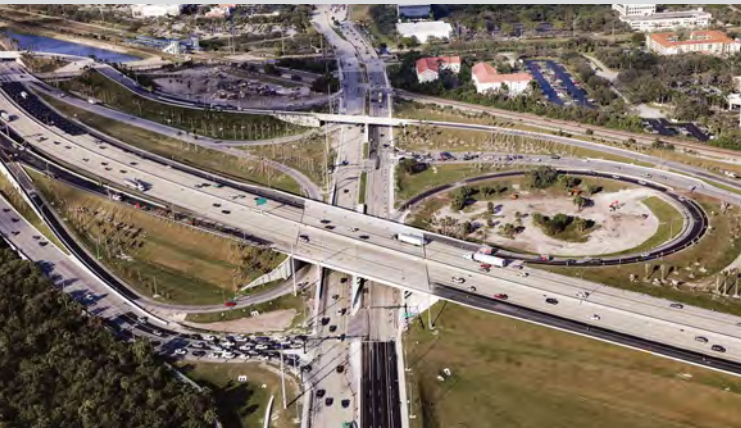
I-95 at Spanish River Boulevard
